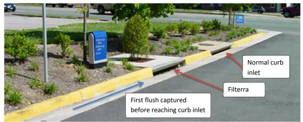
Figure 1 Typical *Filterra* installation (Picture from *Filterra* website)
